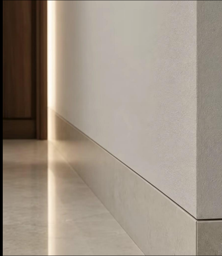
Flush shadow-gap skirting detail
