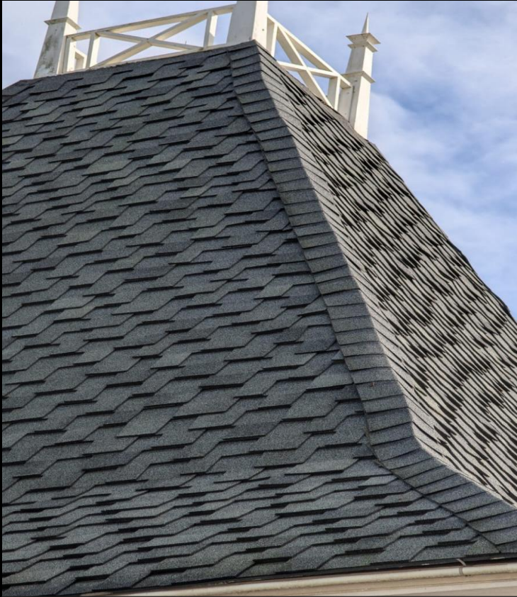
Shingle roof — Maritim Balaclava reference
