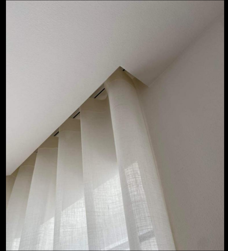
Recessed ceiling curtain track — wave sheers
