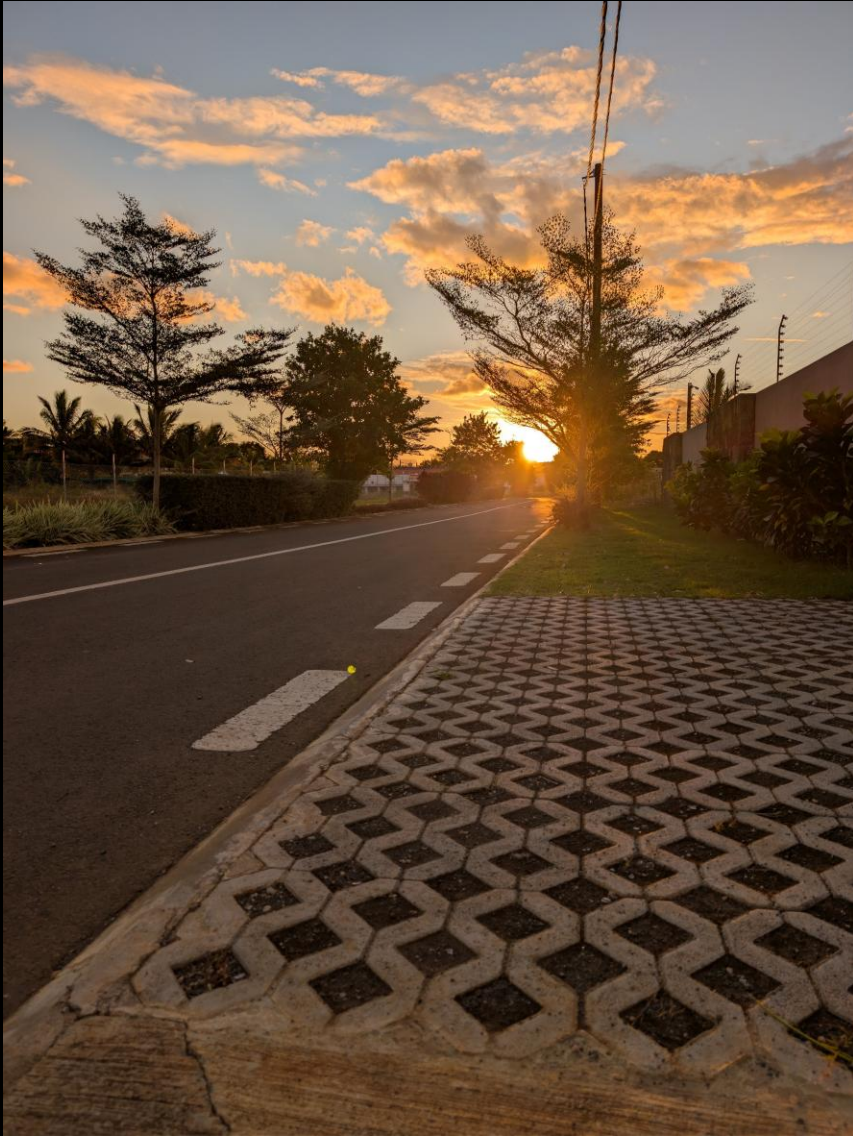
Belgravia Park Built Environment: Private Access Road
