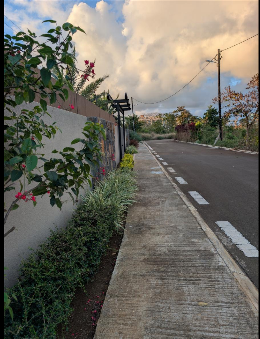
Belgravia Park Built Environment: Private Access Road
